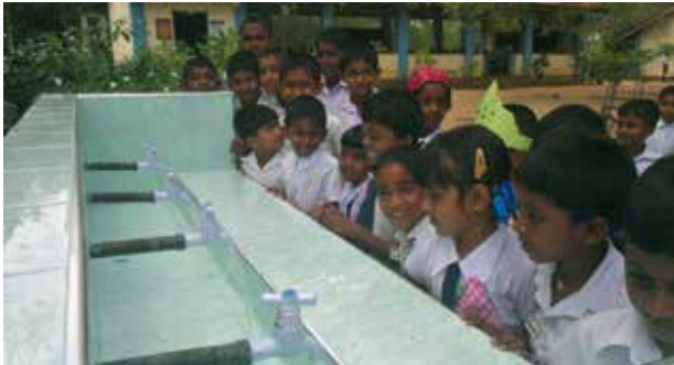
Providing water facilities by Chilaw Branch
